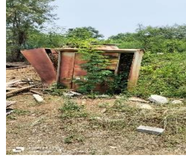
Electrical panel board
