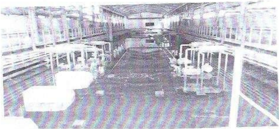
Blast furnace Pump House Water logged
