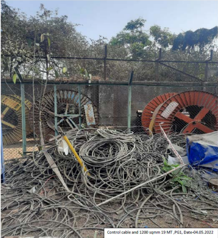
Control cable and 1200 sqmm 19 MT ,PG1, Date-04.05.2022
